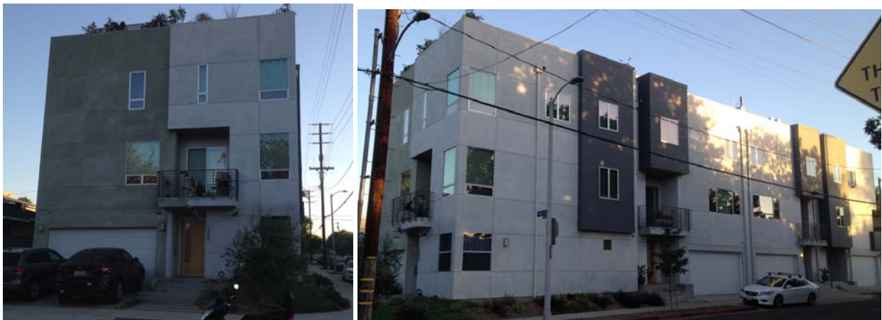
Missouri/Stoner project: Design is blocky with all stucco and no stepbacks or articulation (“logistics center” or “warehouse” school of design)
