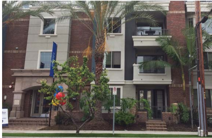
11900 Idaho Ave. Good design units on the ground floor (not parking) with front doors facing The sidewalk with direct connection.
