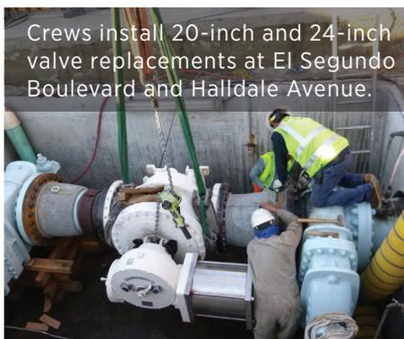
Crews install 20-inch and 24-inch valve replacements at El Segundo Boulevard and Halldale Avenue.
